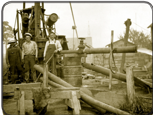
Tapping into the groundwater, as a means of supplementing decreasing supplies, ca
