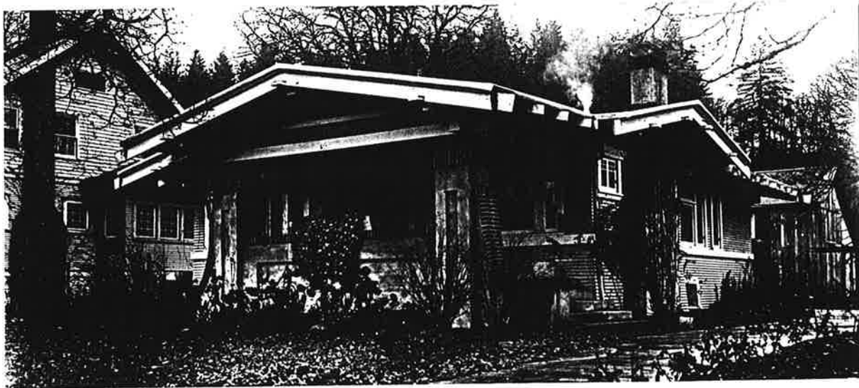
One of Silverton's many Bungalow style homes on Coolidge Street, built in the late 1910s. (Courtesy of Oregon Historical Society, Neg. no.: OrHi 93066.)
