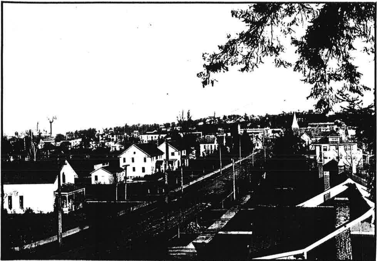
This 1931 scene of apparent prosperity, depicting large homes on West Main Street with smoke from the Silver Falls Timber Company rising in the background, gives little hint of the troubled times ahead for Silverton at the depths of the Great Depression in 1933. (Courtesy of Oregon Historical Society, Negative No.: CN 006763)
