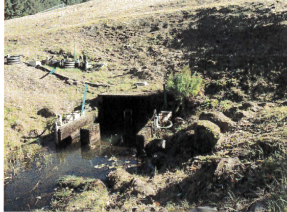
Low level outlet, toe drains, weirs
