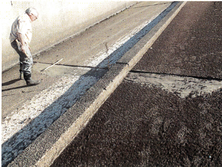
Spillway repair work
