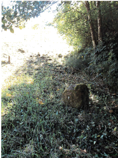
Wet spot below toe
