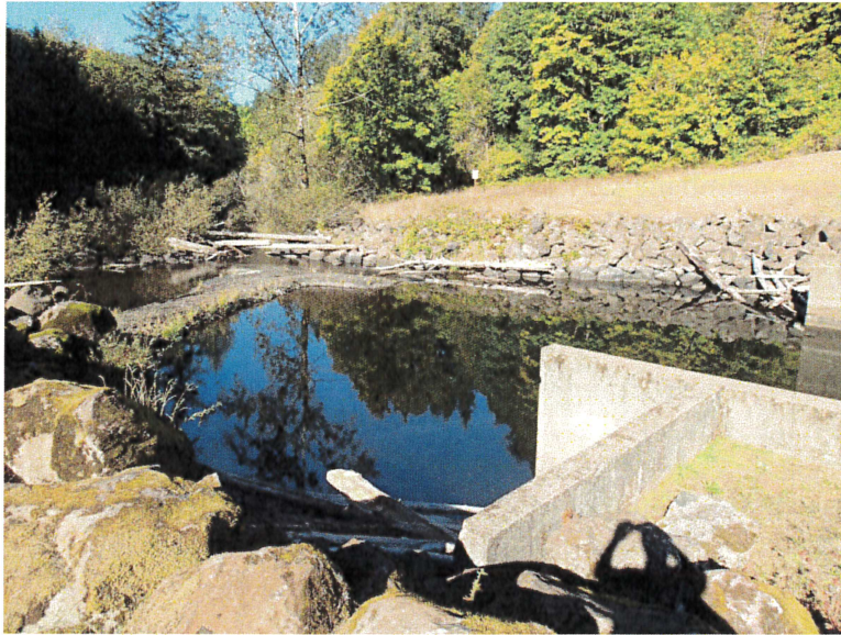
Logs accumulating in stilling basin
