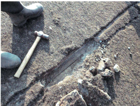
Cracking around slab joints and quick repair
