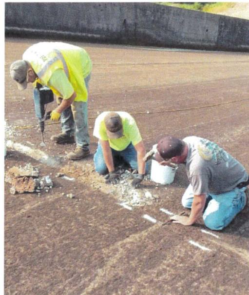
Cracking around slab joints and quick repair
