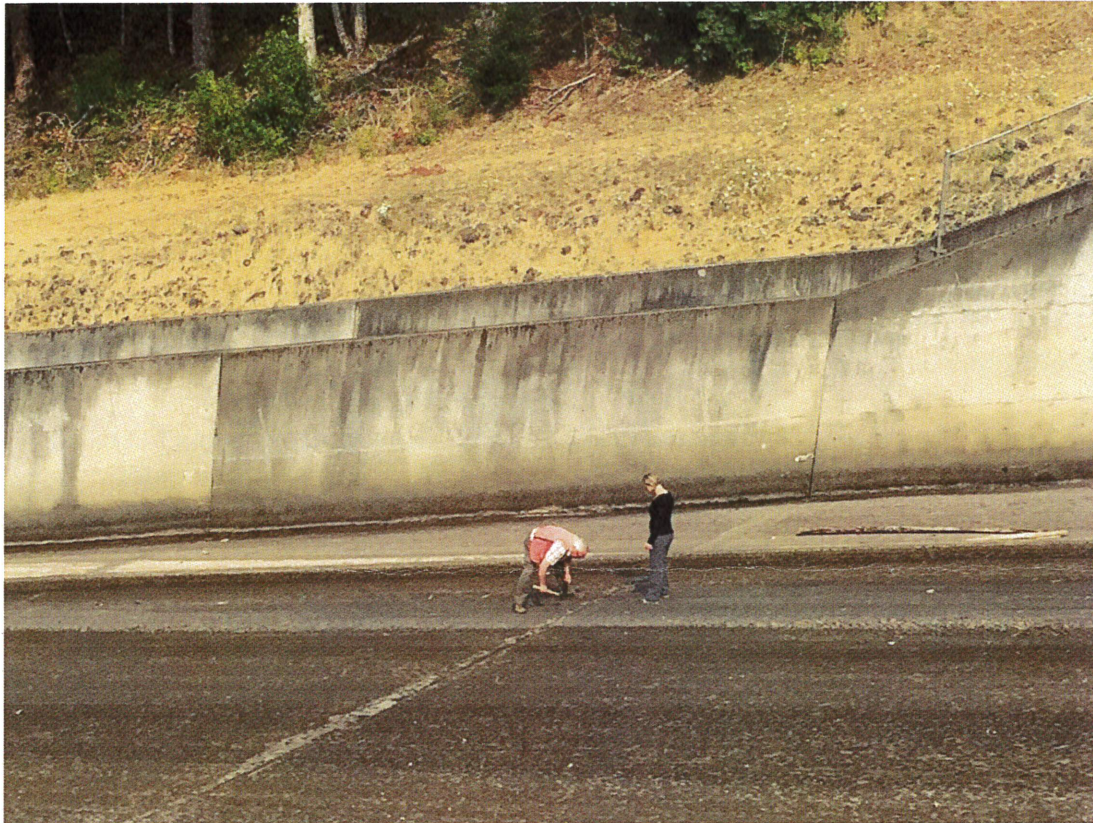
Inspection of the patched concrete repairs
