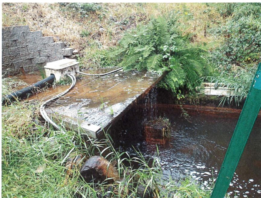
Low level outlet structure
