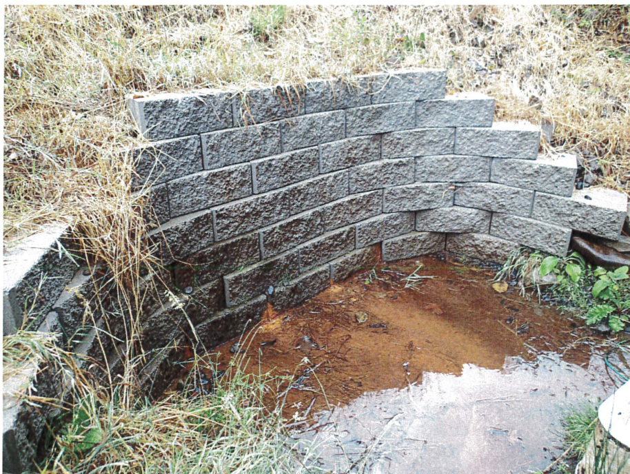
Repaired area of seepage above outlet
