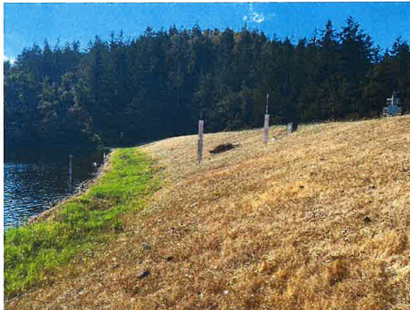
Upstream face of the embankment showing well-kept ground cover
