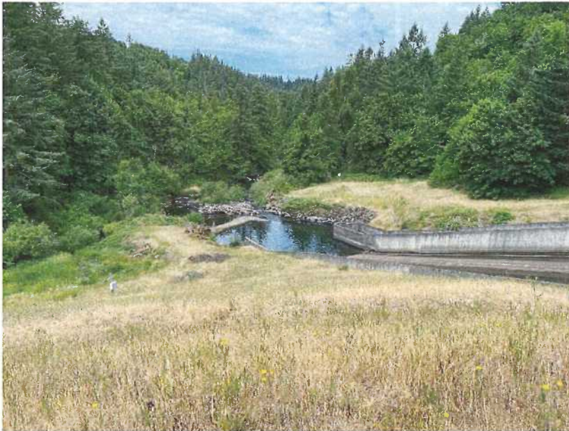
Downstream face of dam and spillway stilling basin
