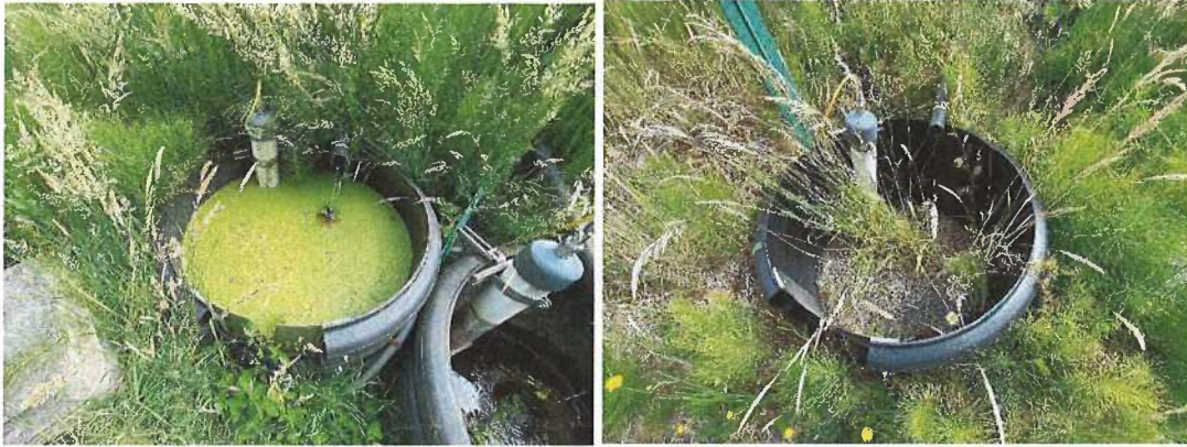
Two of the weirs on site
