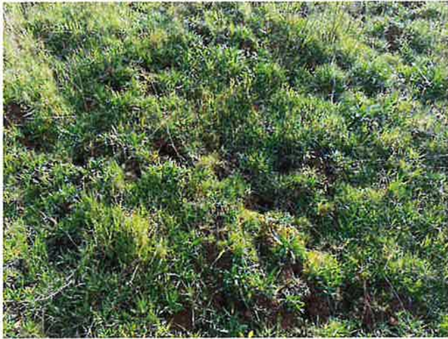
Large area of burrows across downstream face
