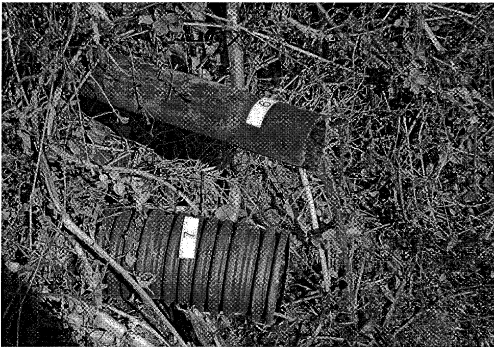
Figure 1c. Pipes 6 and 7 with 6 flowing light and 7 barely flowing.
