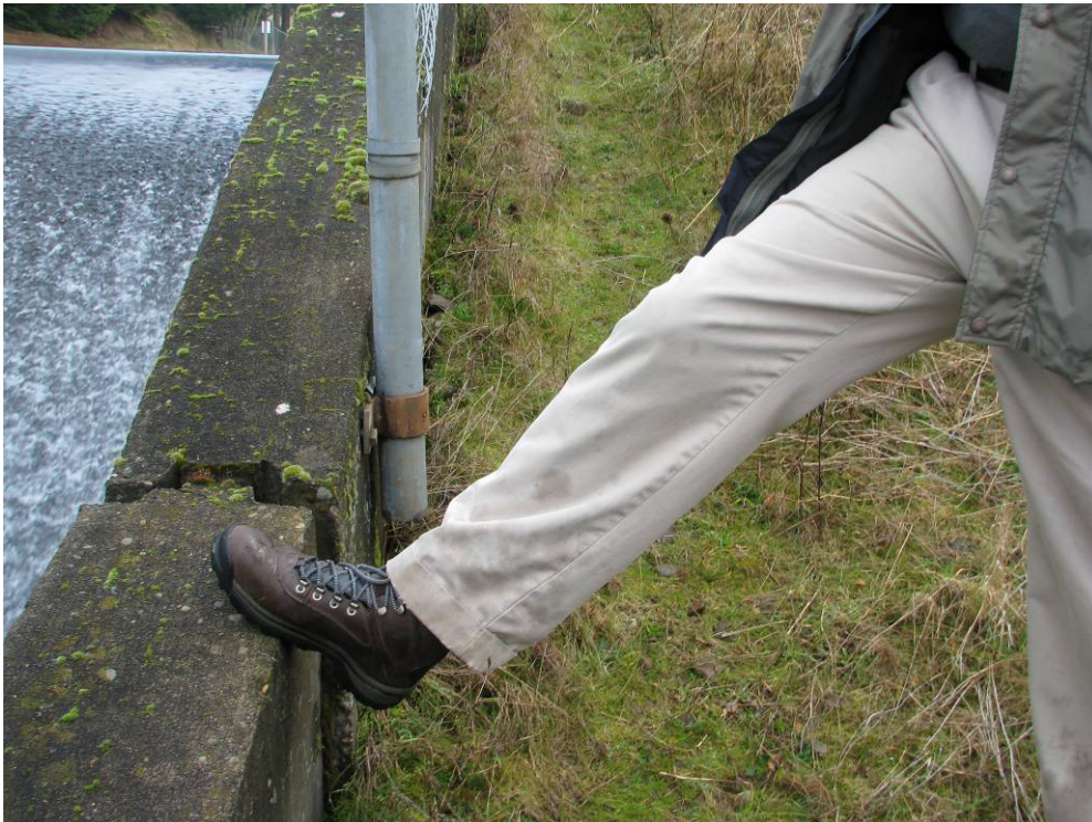
Figure 4. Joint movement in past but stable no movement when compared with other photos.
