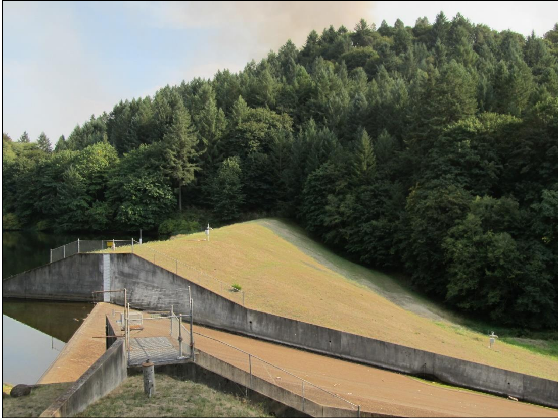
Figure 6-1. Silver Creek Dam crest (looking south)
