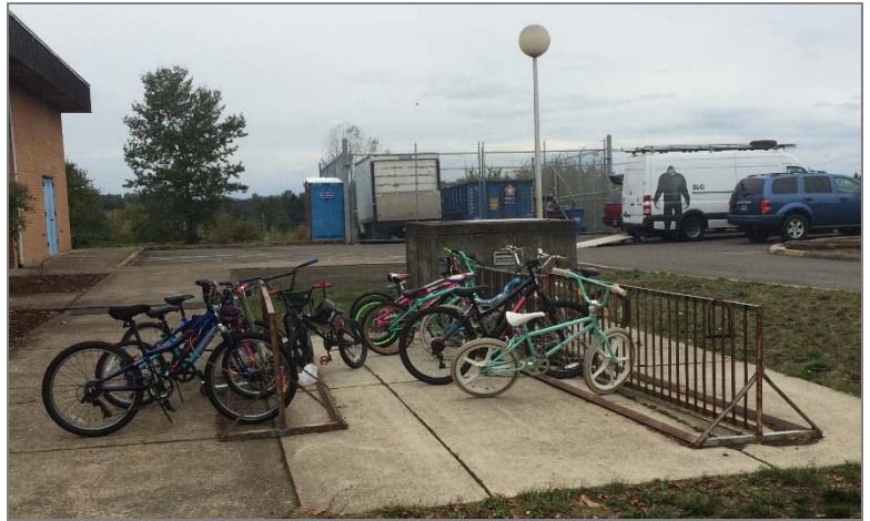
Bicycle parking is relatively well-used but is an older "toaster" style of rack, which does not support the bicycle securely while it is being locked up.
