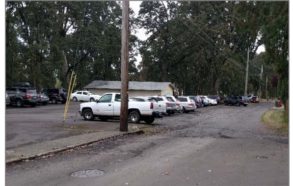
The sidewalk ends at the north school parking lot on Church Street, and vehicles enter, exit, and park in the lot irregularly, causing conflicts with people walking.
