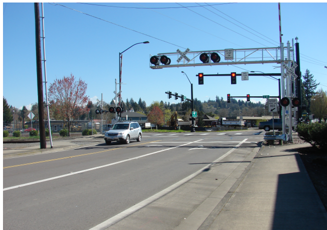
Figure 17: Rail crossing at C Street/Water Street
