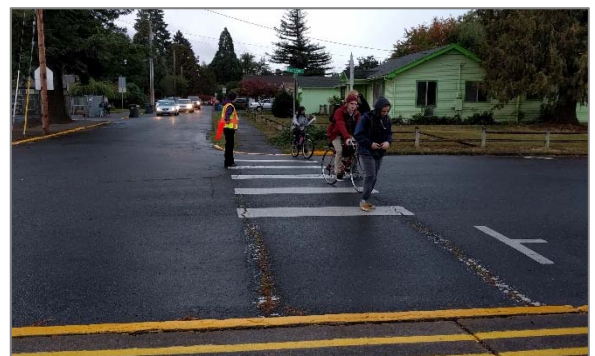
The main school crosswalk across Schlador Street and Brown Street lacks ADA-compliant curb ramps on both ends.
