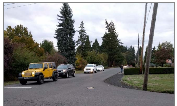
Western Avenue is an important connection to the overflow student parking lot, but it lacks sidewalks.
