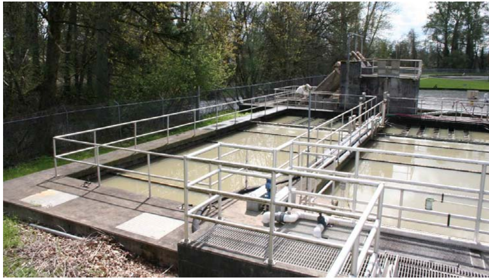
Figure 7-15: Silverton WWTP Primary Clarifiers
