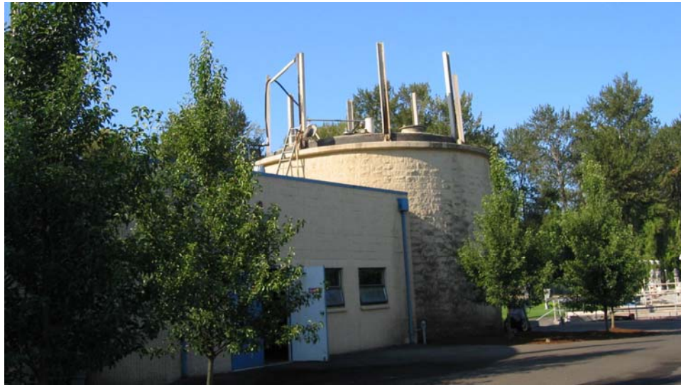
Figure 9-15. Silverton Anaerobic Digesters and Digester Control Building
