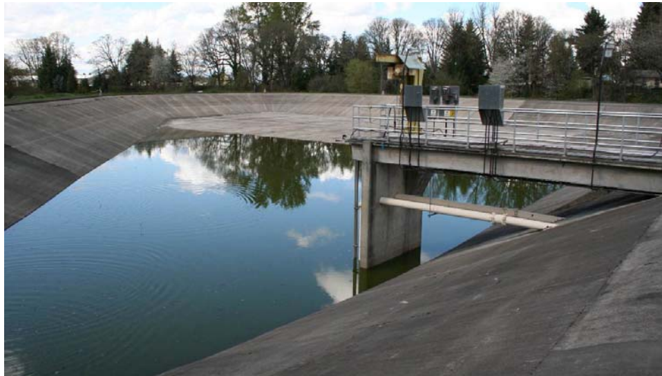
Figure 7-23: Silverton WWTP Flow Equalization Basin
