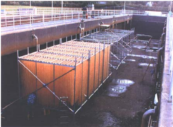
Figure 9-1: Examples of IFAS Hybrid media system
