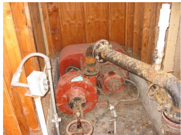
Figure 7-16: Primary Sludge Pump Shelter (Tan Walls with Blue Roof) (Left) and Primary Sludge Pump (Right)
