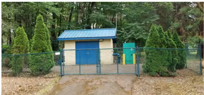
Edison Road Booster Pump House
