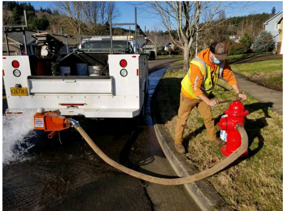
City of Silverton Public Works employee flushing a fire hydrant
