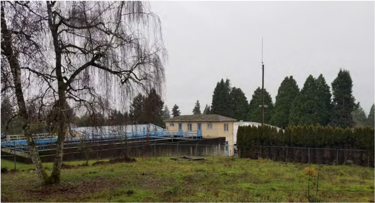
Silvertown Water Treatment Plant
