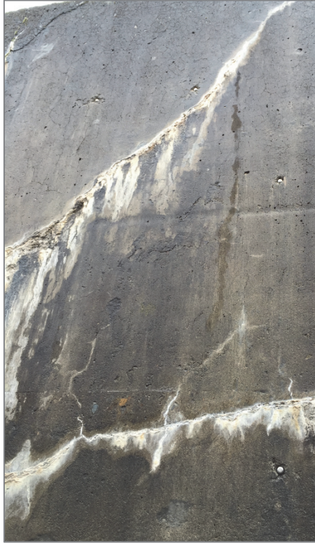
Exhibit 3.9 – Cracked Concrete Leaks
