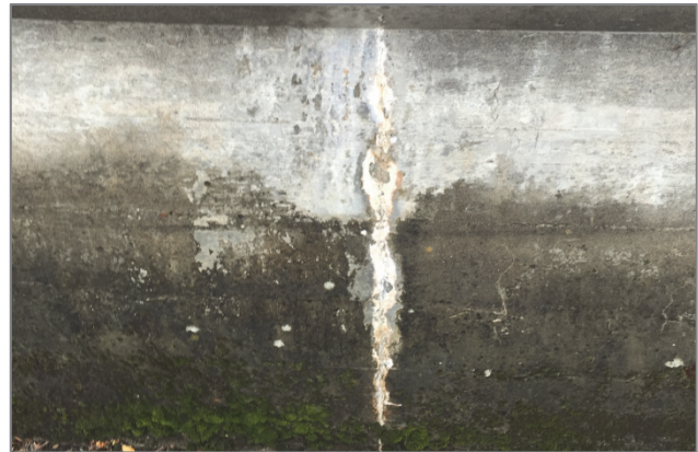
Exhibit 3.9 – Cracked Concrete Leaks
