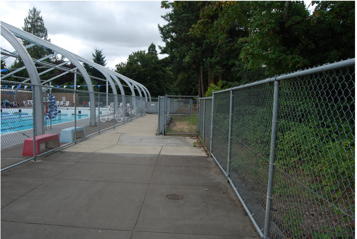
Location of original surge tank
