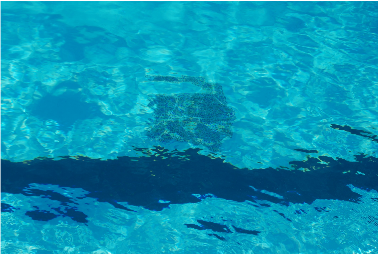
Main Drain Grate
