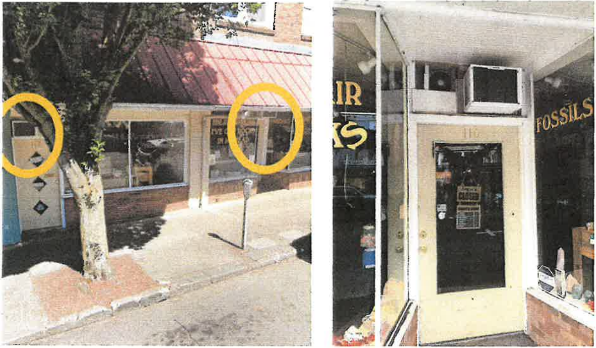
Figure 3C: showing 2 A/C wall units that protrude from the building.
