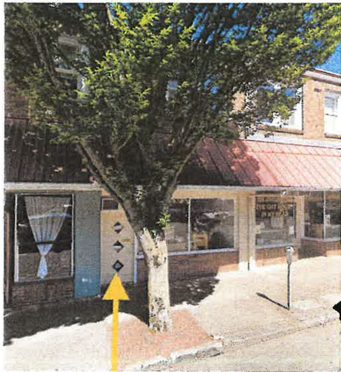
Figure 3D: showing exterior door that does not match current facade. We plan to replace this non functioning door with a glass commercial door that meets ADA requirements
