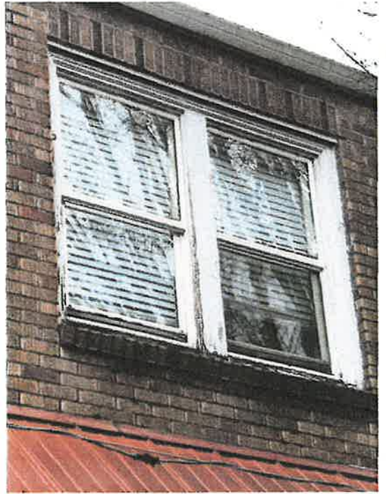
Figure 3A: showing paint peeling from windowsills on upper level of building.
