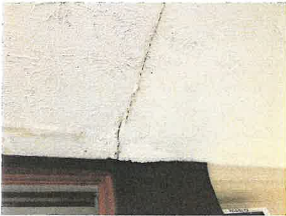
Figure 2A: Showing leaking soffits that are bubbling and deteriorating from water damage under awning.
