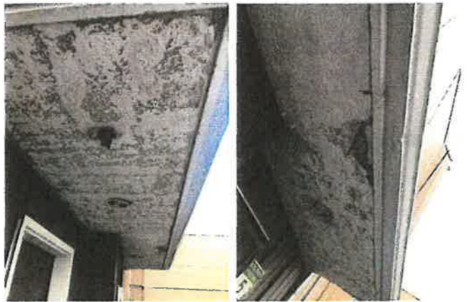
Figure 2A: Showing leaking soffits that are bubbling and deteriorating from water damage under awning.
