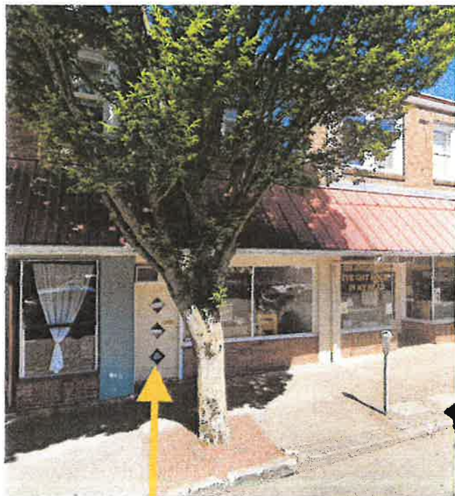
Figure 3D: showing exterior door that does not match current facade. We plan to replace this non functioning door with a glass commercial door that meets ADA requirements
